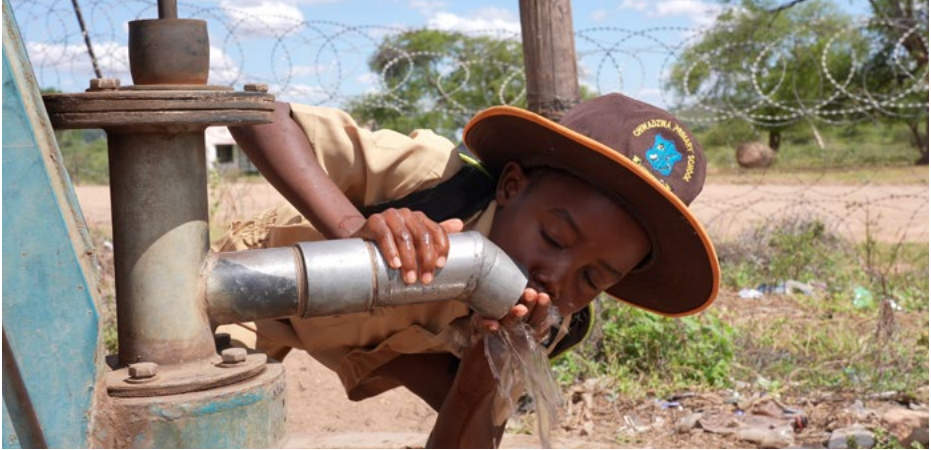
A Chiadzwa Primary School student quenching his thirst at a rehabilitated community borehole in Chiadzwa.
